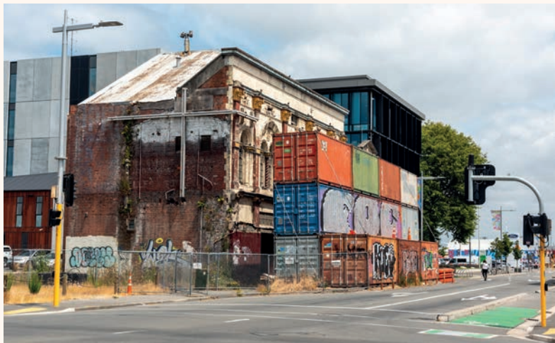
← New legislation following Canterbury earthquakes requires URM buildings in New Zealand to be strengthened or demolished
