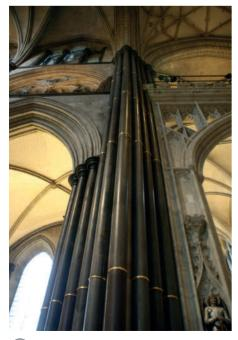
Stability in any large masonry structure is time dependent. Even if the structure is built with tight joints and so negligible creep, the foundations will creep if the stress gets a bit high and this will induce rotations that reduce (however slowly) stability. The bent columns in Salisbury Cathedral (Figure 1) show this action in progress.
