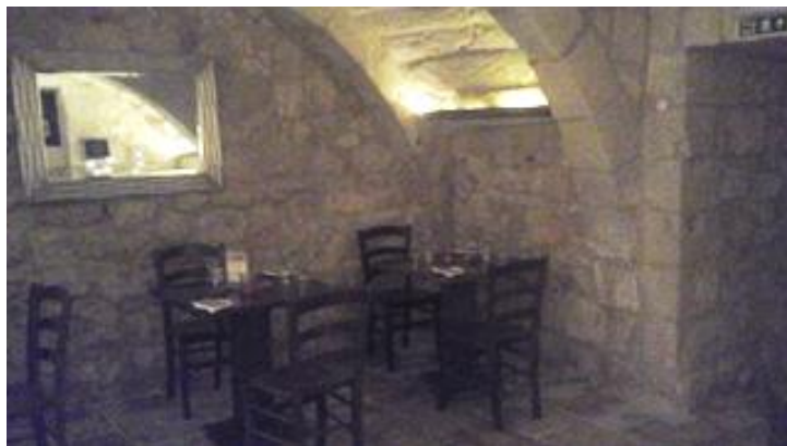
Figure 5: this basement construction in Rabat probably pre-dates the overlying 16 th century palatial construction. Rubble infill masonry abuts onto the street walling, whilst the supporting masonry arch quoins are formed in ashlar masonry. 1m masonry slabs span onto the arches, whilst flooring is in tal-qawwi flagstones. (SOURCE: Author)
