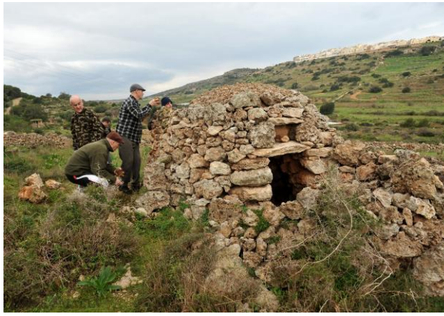
Figure 3: A corbelled hut (girna), constructed in rubble masonry of locally sourced UCL, being maintained by hunters. The same construction is utilised as in the dry stone walling, as separating the fields [18]
