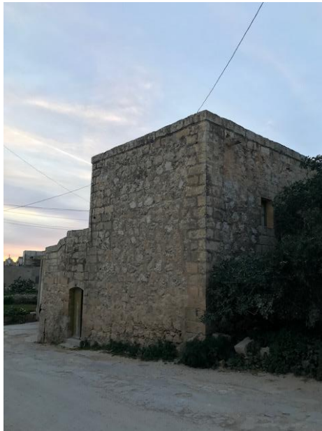
Figure 4: Construction in Gozo, note rubble infill walling with ashlar at the corners, together with the top string ashlar course. (SOURCE: Author)
