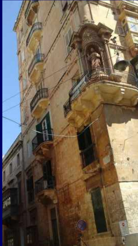
An 8-storey high apartment block constructed, as 1908 in compact globigerina limestone, Valletta
