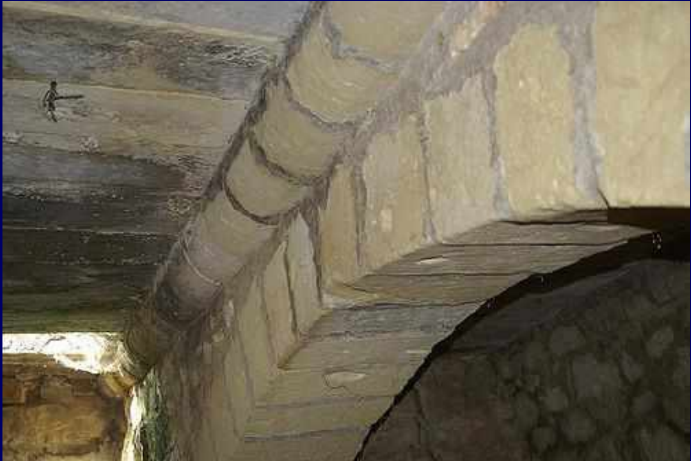
Xorok supported by arch construction at 1m centres.
