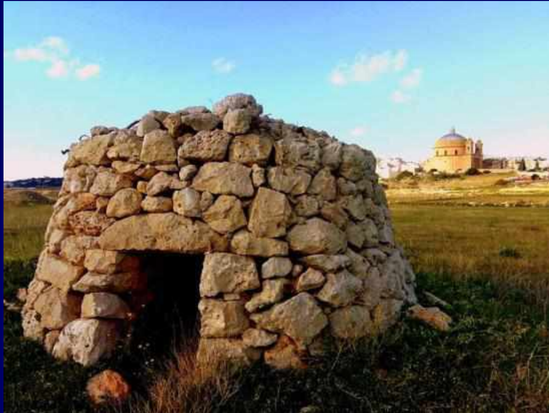
A corbelled hut (girna), constructed in dry stone masonry of locally sourced UCL – not common in Southern Italy.
