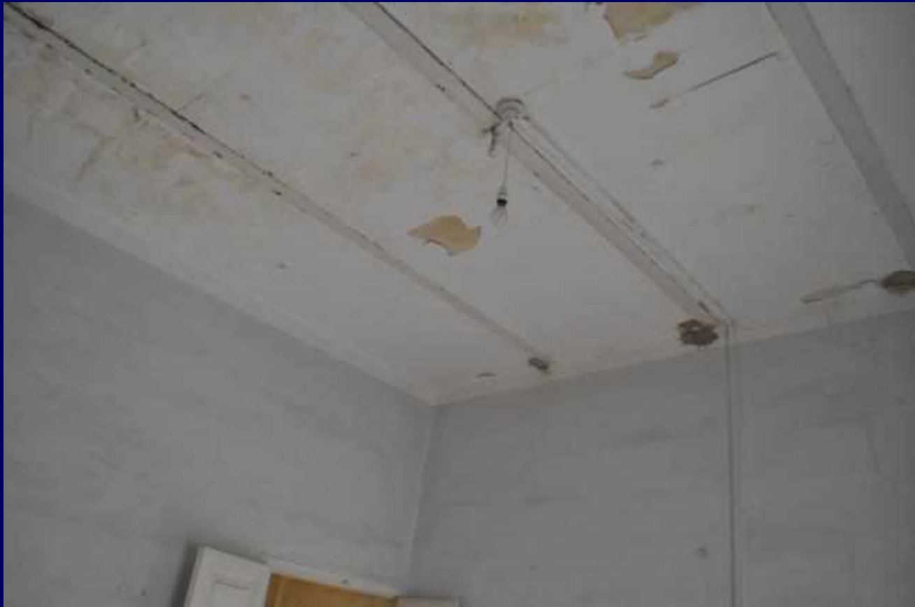
A typical townhouse soffit from the British Period with embedded steel joists – note flaking plaster & rusty joists.
