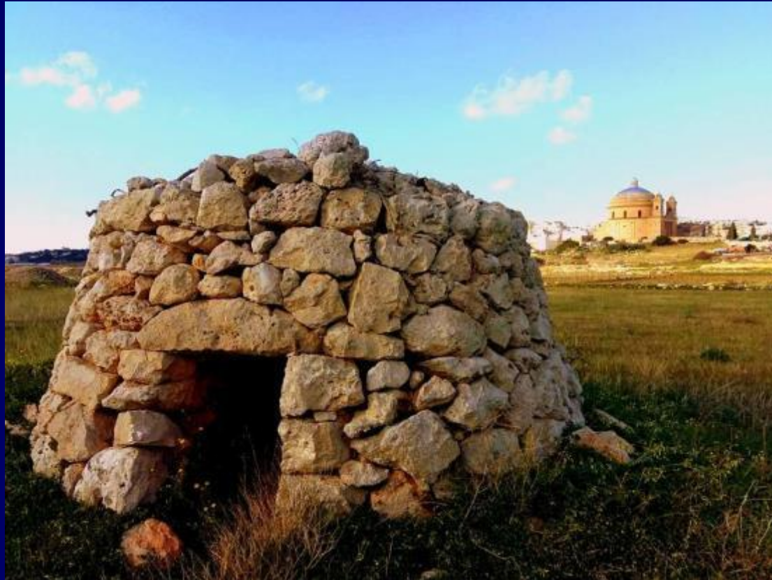
A corbelled hit (girna), constructed in rubble masonry of locally sources UCL
