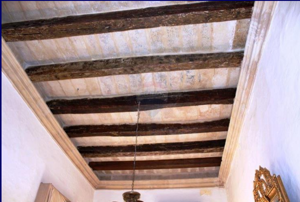
A typical timber joist ceiling
