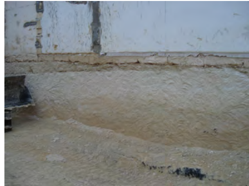
Figure 12.2: Use of hydraulic milling cutter.
