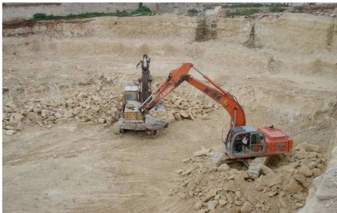
Figure 3: Hydraulic hammers in operation at Marsascala site
